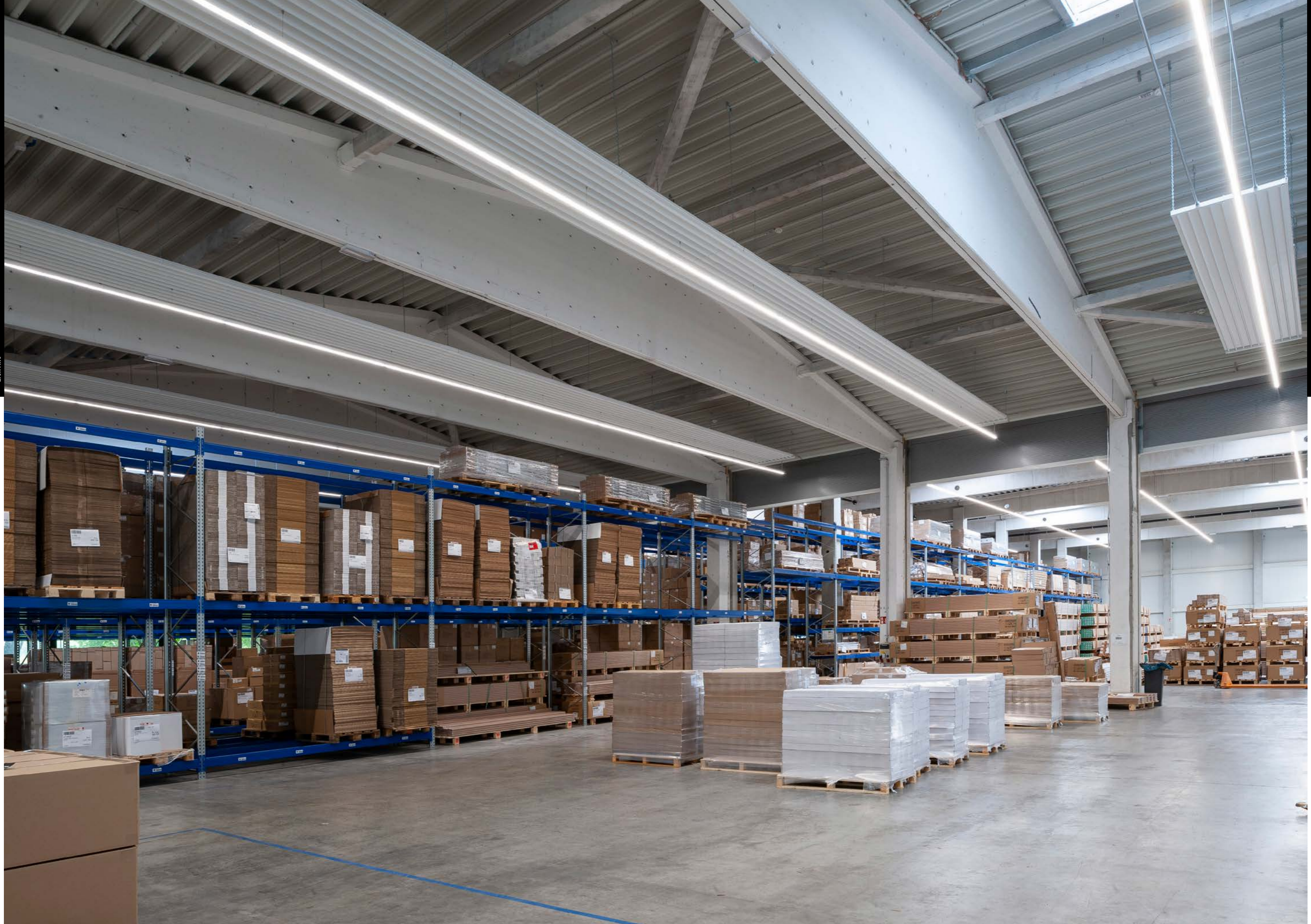
Warehouse: 3500m 2 , mounting height: 6m, Installed Light power: 300lx, Trail Light insert medium beam (60°), High Efficiency (HE), DALI
